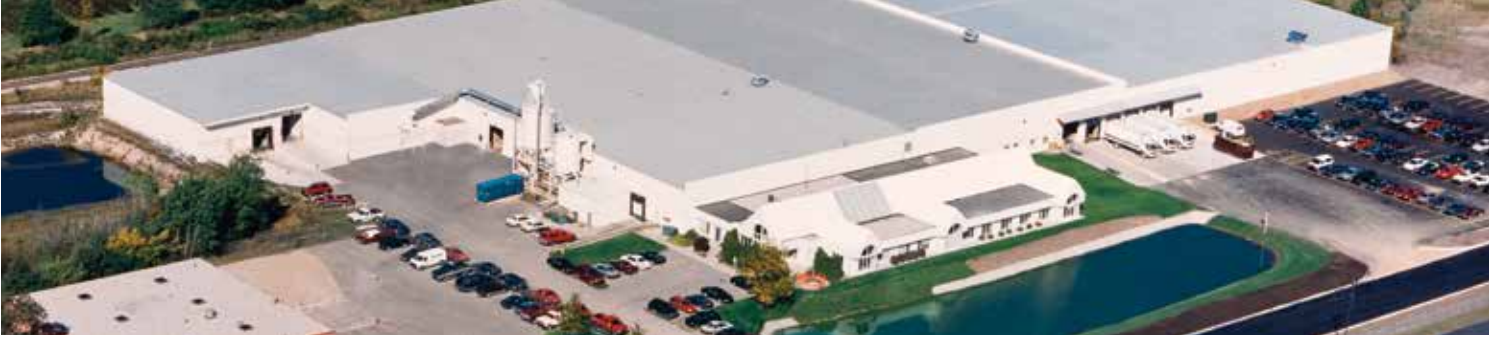
Our 187,000-sq. ft. manufacturing facility in Holland, Michigan.
